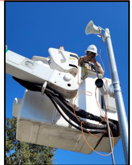
Rossville camera system installation
