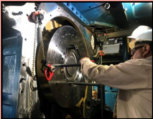
Removing Vibration Damper
