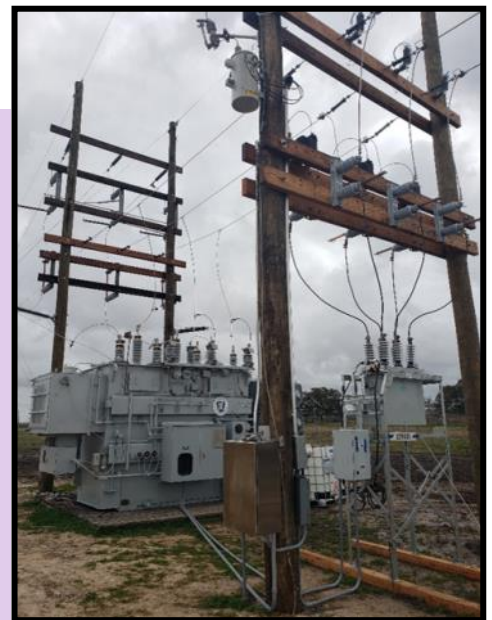
Rio Colorado temporary equipment installation
