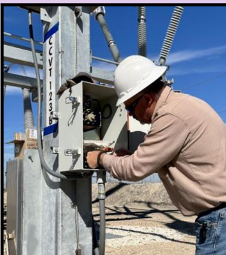
Gary Cowey wiring a line tuner cabinet
