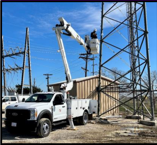
Jeff Carpenter installing an antenna at El Campo
